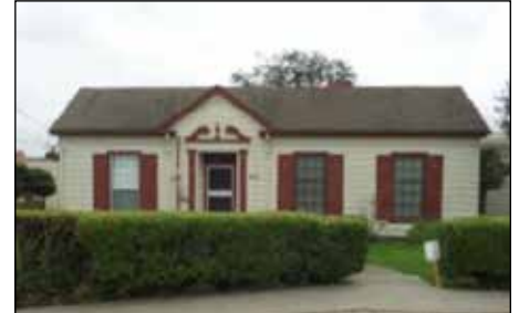
The Soledad House in Salinas is Interim's original crisis residential facility.
